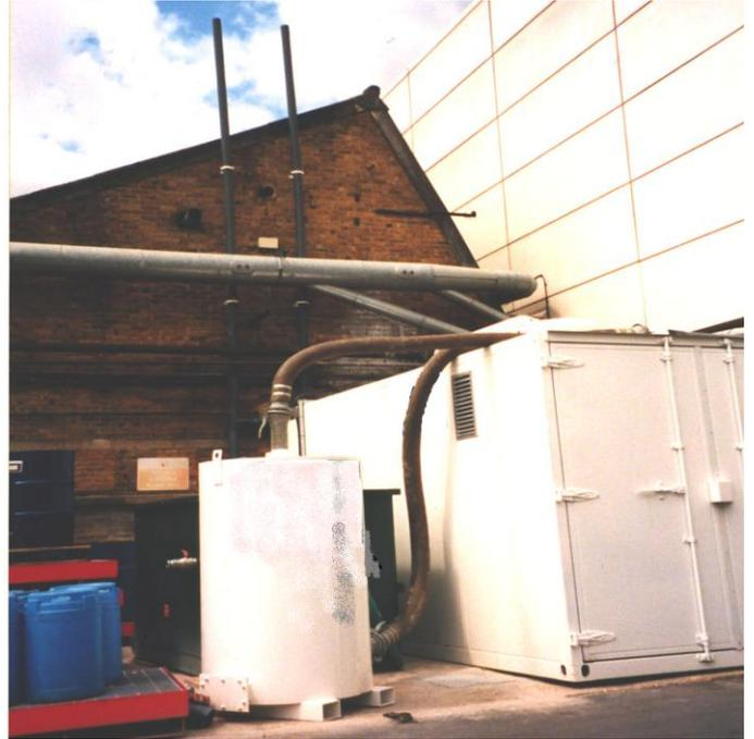
The vacuum extraction system exhausts through an activated carbon filter to minimise emissions to the atmosphere. In total over 2,500 kg of VOCs were removed by the treatment process.
